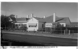
Somers House, 225 Beach Road, Blackrock, Vic
