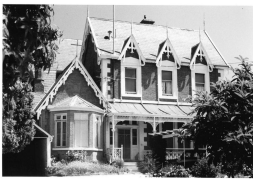
Geelong. Hawthorne St. Mary's Hostel 39 Skene St.
