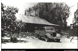
Griffiths House - building new boys dormitory
