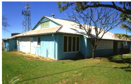
Pine Creek Repeater Station
