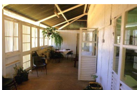
Pine Creek Repeater Station
