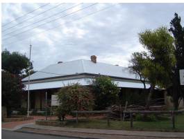
New Roof [former site of Forrest Lodge]
