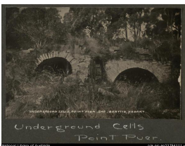
Underground Cells at Point Puer
