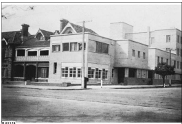
Exterior view of 'Queen's Home'
