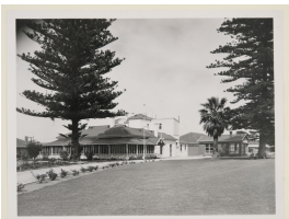
Seaforth Home, Entrance
