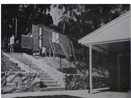
Woorabinda Campsite under construction
