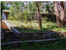
Former Hostel Building at Lake Woorabinda
