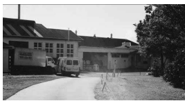
Holy Cross entry/despatch section of laundry building
