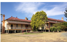
Original buildings, Riverview
