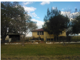
House, Darling Downs Correctional Centre
