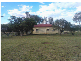
House, Darling Downs Correctional Centre
