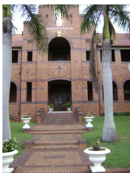
Main Entrance of Nazareth House Wynnum North
