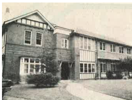
The former Carramar Hostel, Turramurra
