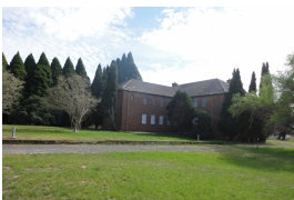
Challoner Cottage viewed from Bong Bong Road
