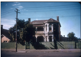
Presbyterian Sisterhood Home - the building from the street
