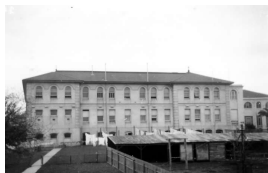
St Anthony's Home, Kew, buildings [rear]
